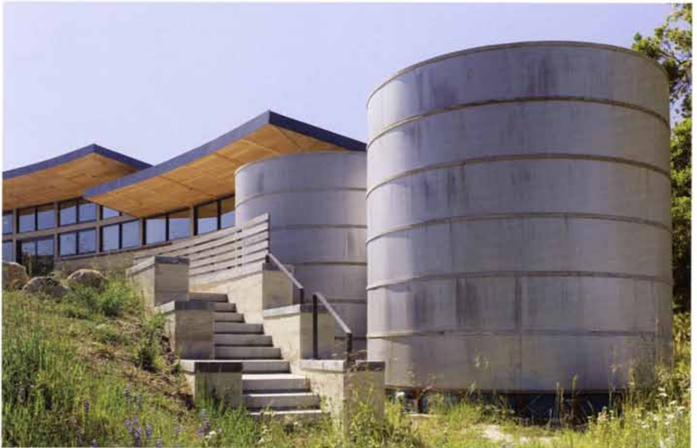
Right: Walls built with earth excavated from the site.
