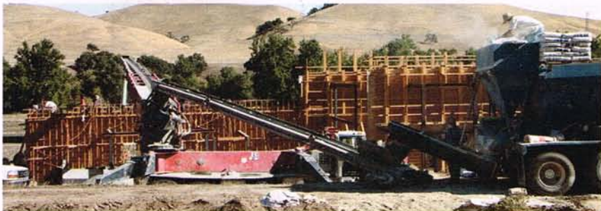
Ingredients were combined in a volumetric mixer and conveyed to the forms by a belt truck.
